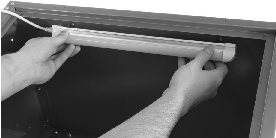
Figure 10 : Montage tube fluorescent
